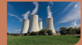
Power & Ash Handling
