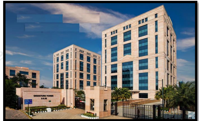
Google Signature Tower, Gurgaon
