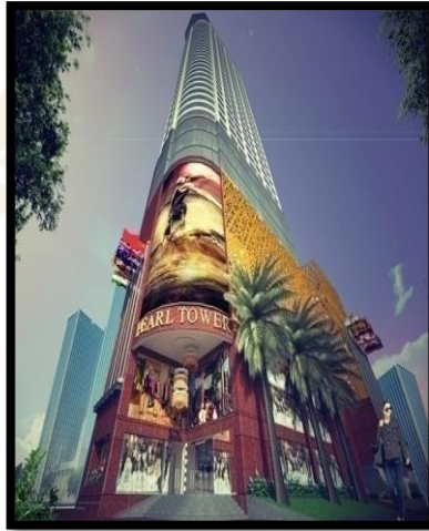
Pearl Tower, Intercontinental Hotel Colombo
