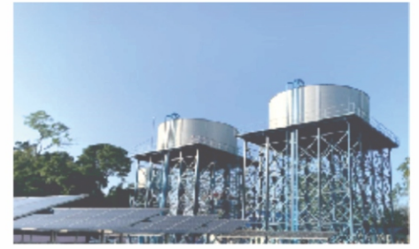
Tank on Staging
